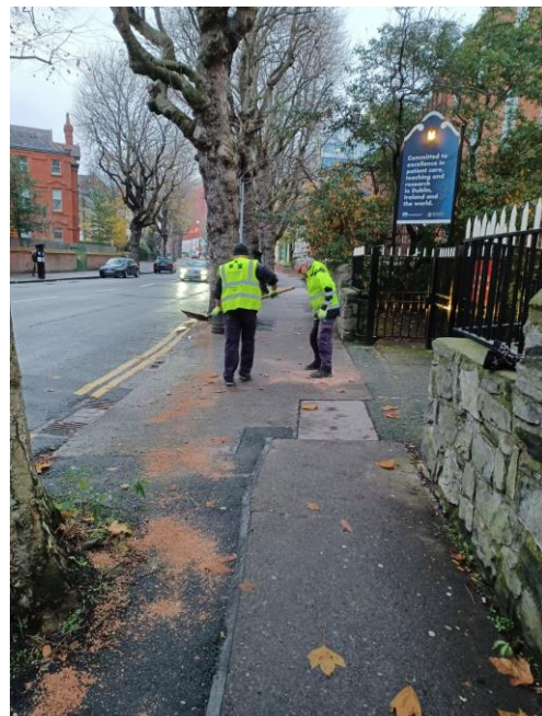
Photograph 8. WMS spreading rock salt by shovel
