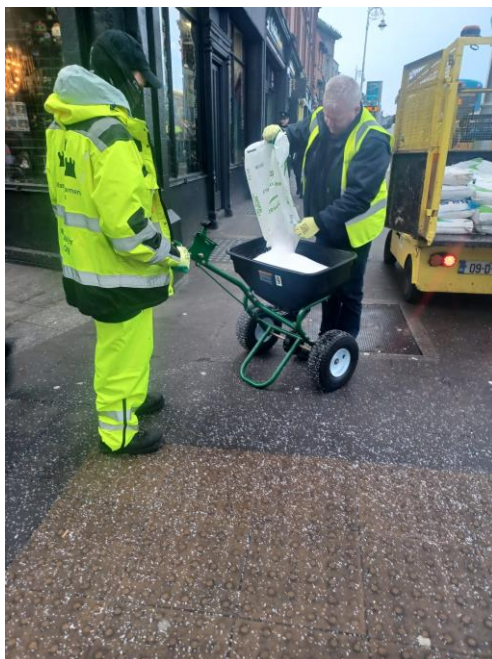
Photograph 7. WMS loading mini-gritter with white salt
