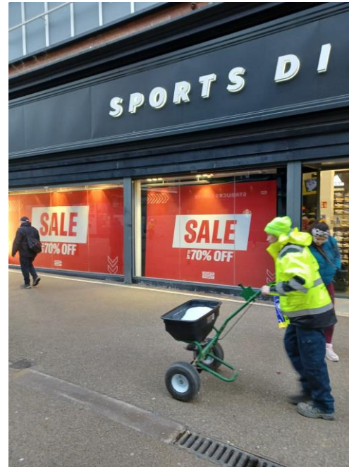
Photograph 6. WMS using mini-gritter to disperse salt
